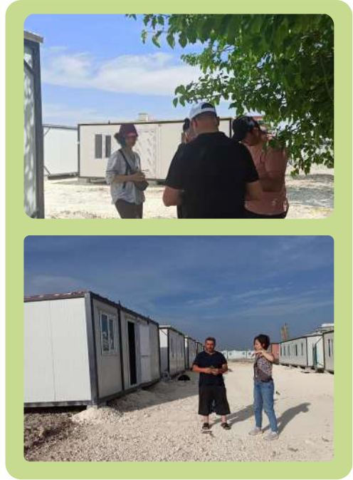
Adiyaman, Eylül 2023, K15 Container Houses Construction Process
